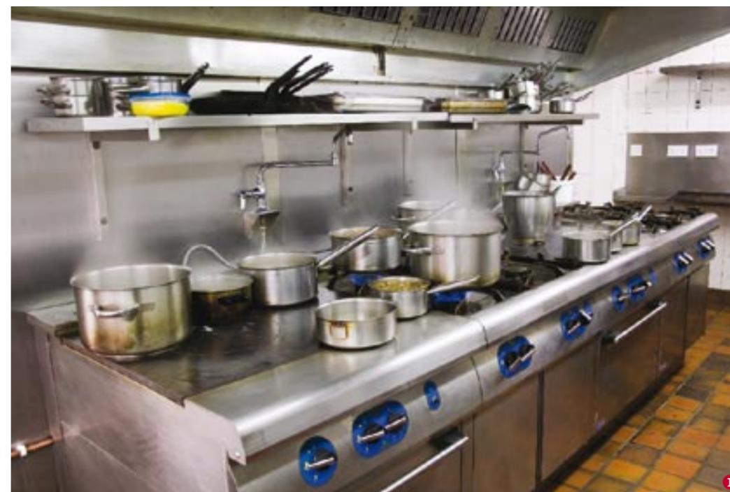
**1** The Bonnet Optimum 900 modular suite is made up of two four-burner ranges and two solid-top ranges with ovens underneath, arranged alternately to provide a section for meat and fish and another for garnish. The 8.8kW and 5.5kW burners feature electronic ignition, and welded tops mean there are no seams to trap debris. A cold-water flush that runs into the drains helps to keep the temperature down and the stovetops clean.
